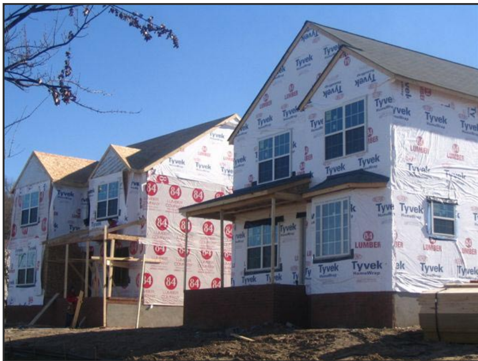
Construction of single-family homes in Fulton is underway
