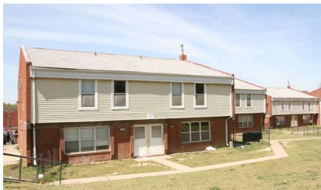
Dove Court Apartments - today
